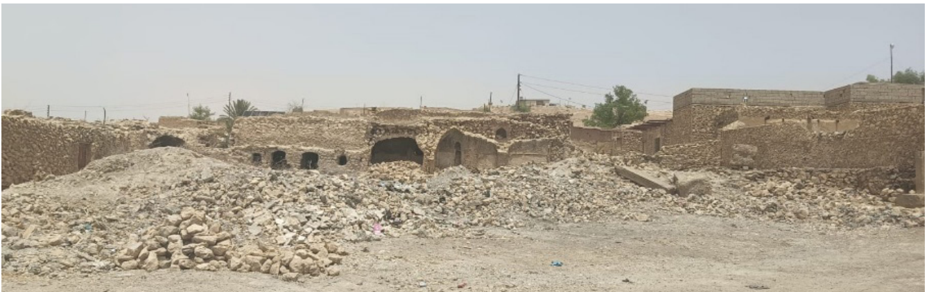
Figure 2 Housing Damage in Sheikh Ibrahim
