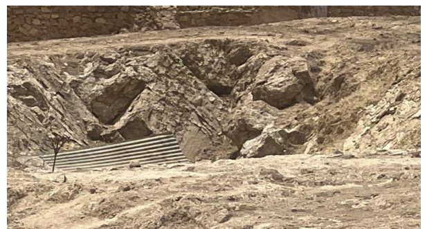
Figure 5 The destroyed well that needs maintenance and cleaning.
